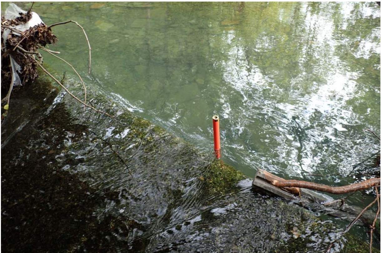
View of the vertical rise from the bottom of the streambed to the floor at the inlet of the south span.
