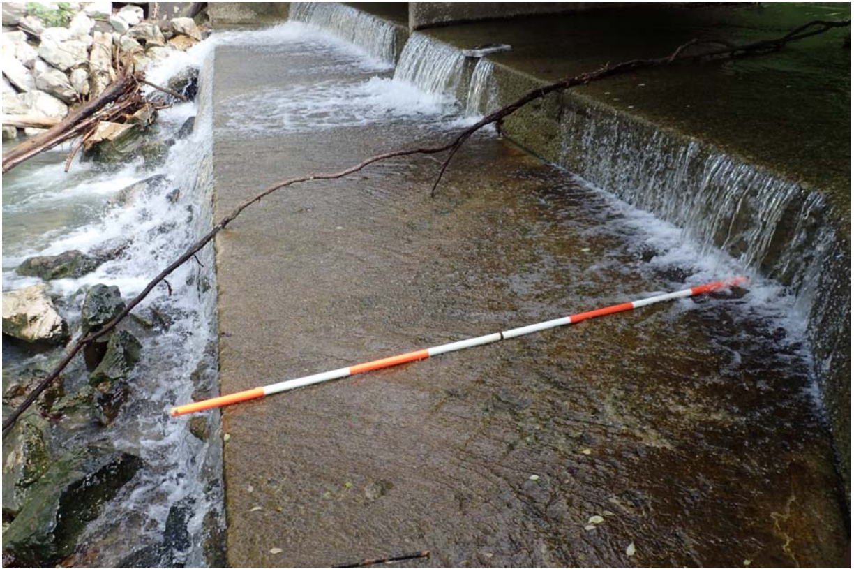
View of the ~ width of the downstream protection apron.
