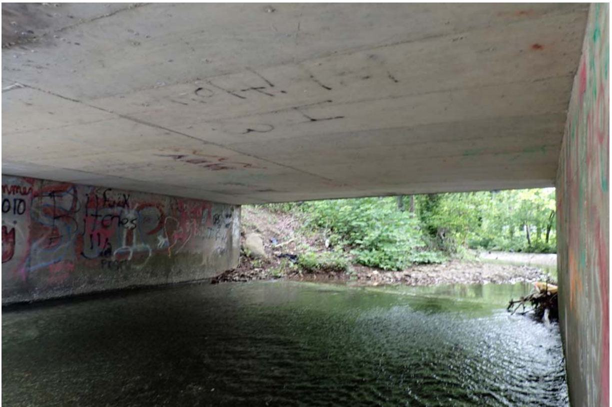
Typical view looking through the north span.
