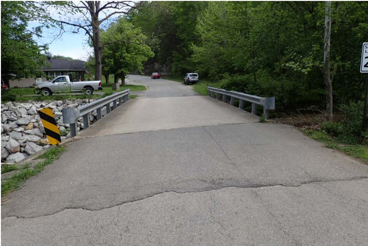
Typical view from the south approach.
