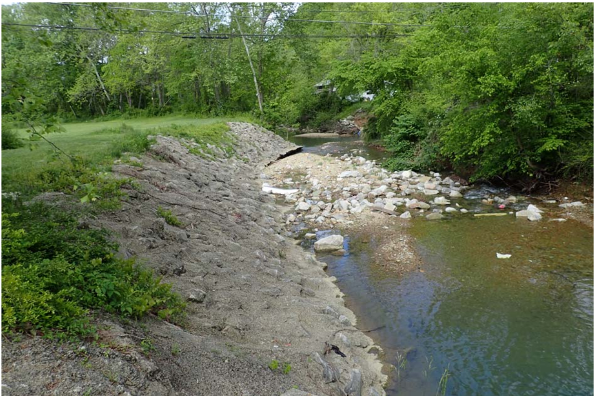
Typical view looking downstream from the south end of the structure.
