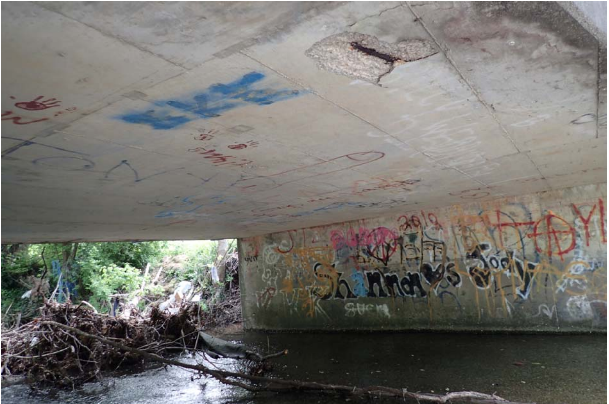
Typical view looking through the south span.
